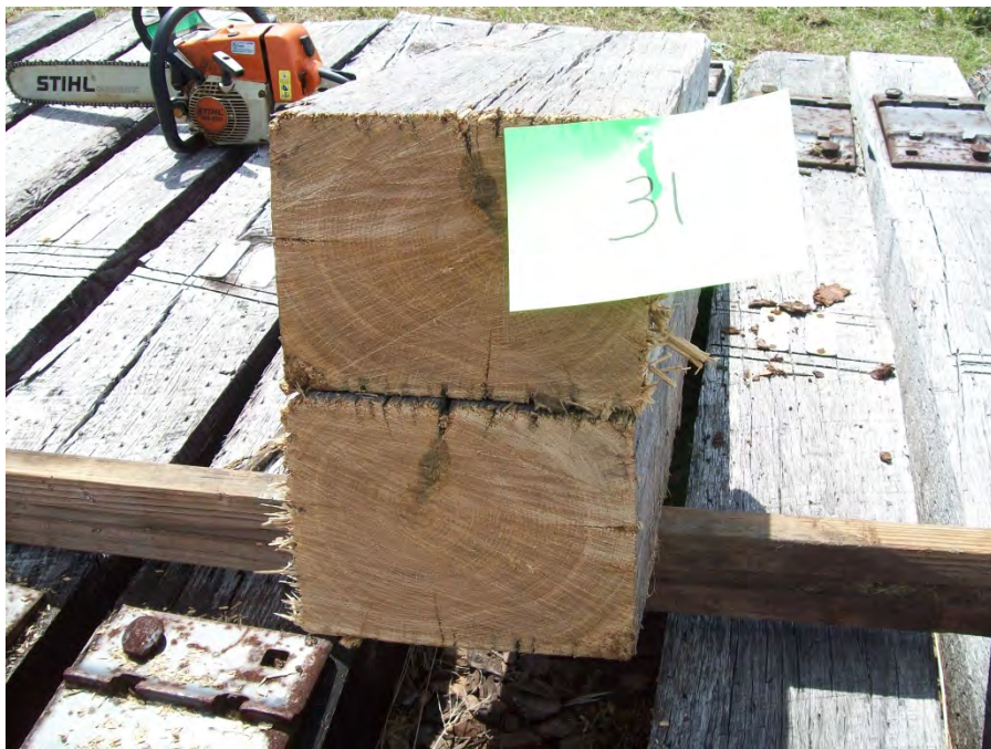
Figure 60 - Tie #31 untreated white oak with decay visible in the sapwood.
