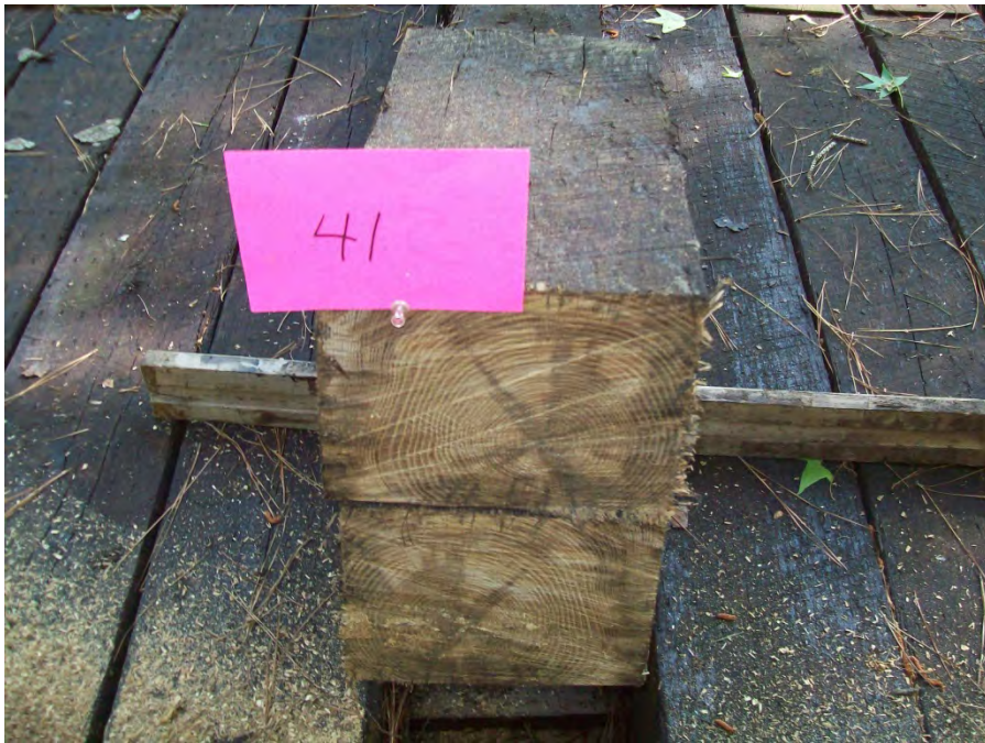
Figure 10 - Tie #41 white oak/borate/creosote 7lbs (Koppers).
