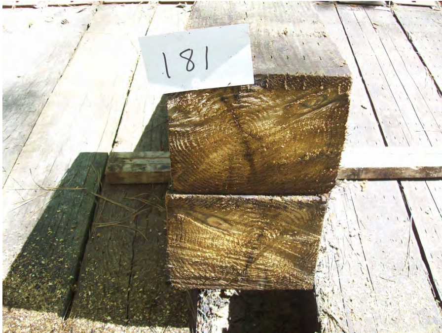
Figure 40 - Tie #181 Douglas fir/P2 creosote (Lonza).
